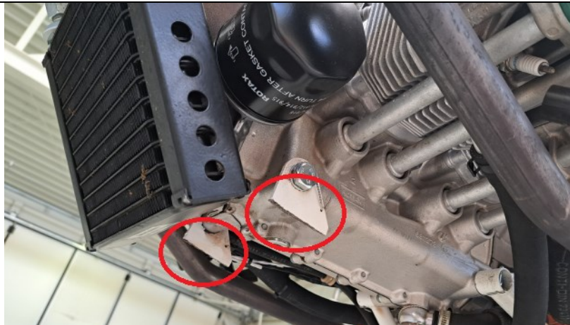
Figure 5 Remaining lugs after loss of ballast
